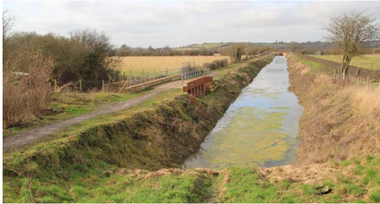
The restored stretch of canal at Chaddington (Doug Small)
