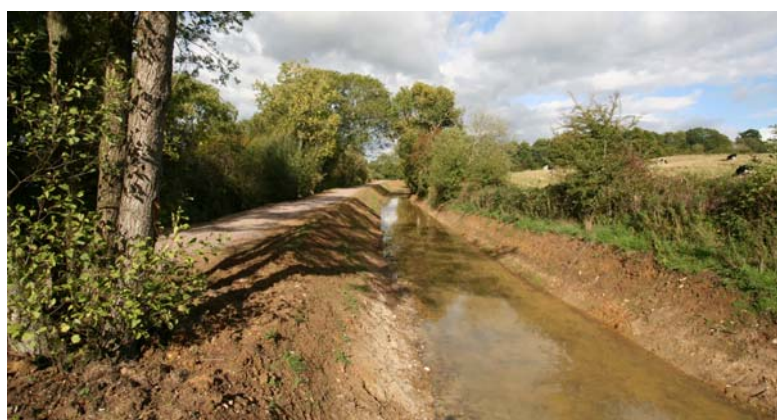
The dredged section at Pewsham (John Minns)
