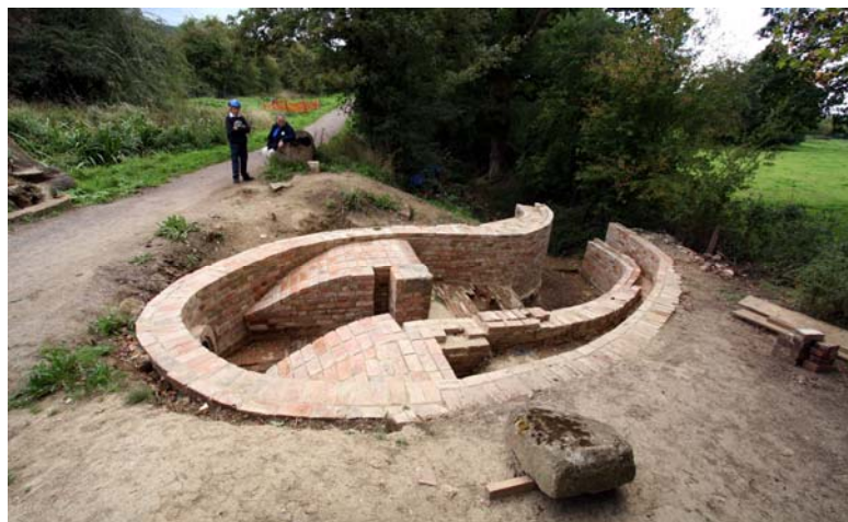
The horseshoe shaped spillweir at Pewsham (John Minns)
