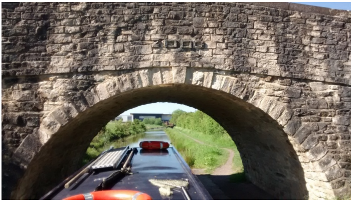
Passing under Beavan's Bridge. Credit: Chris Barry
