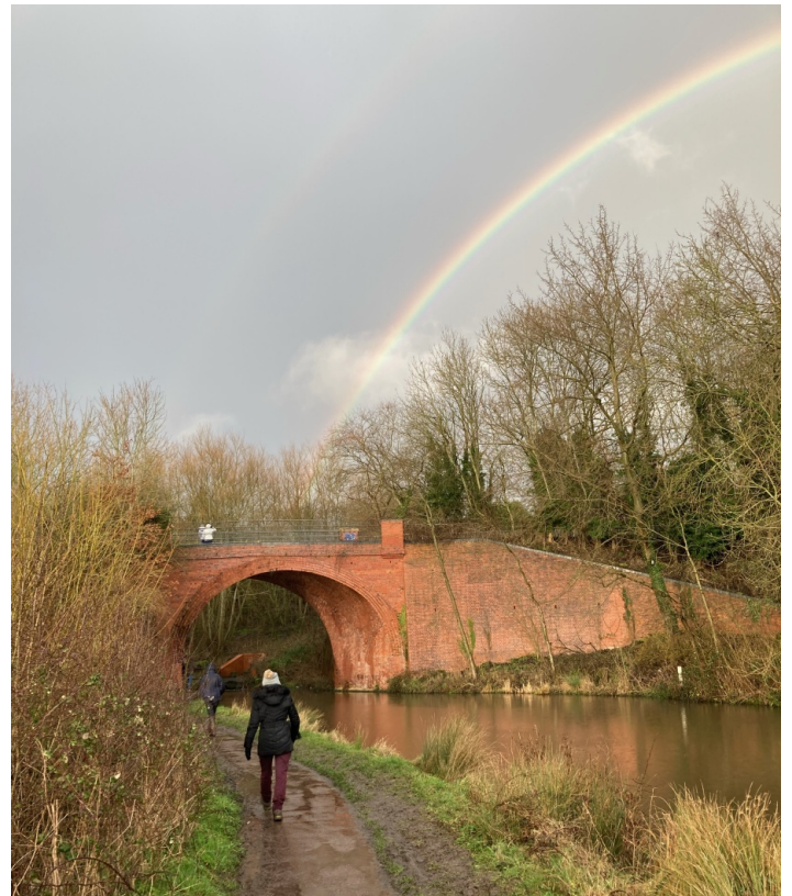
Skew Bridge. Credit: Chris Barry
