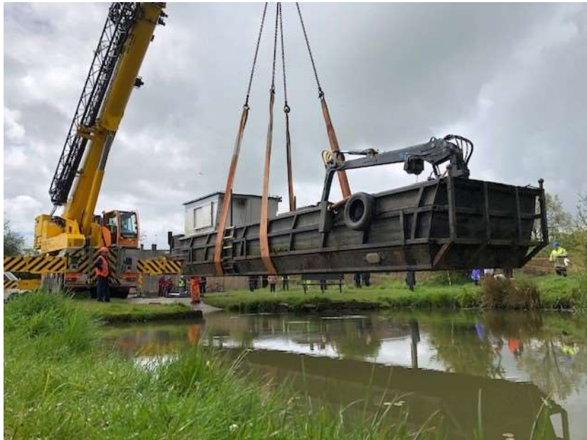
Boat above the water ready to be lowered.
