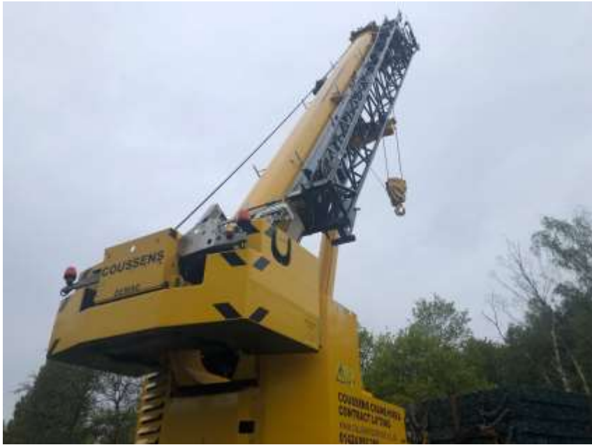
The 100-ton mobile crane in position, 15 th May.
