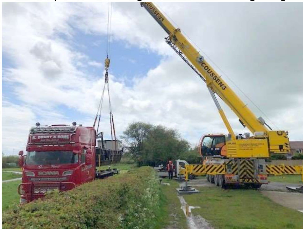
Crane in place beside slipway, lifting boat from lorry.
