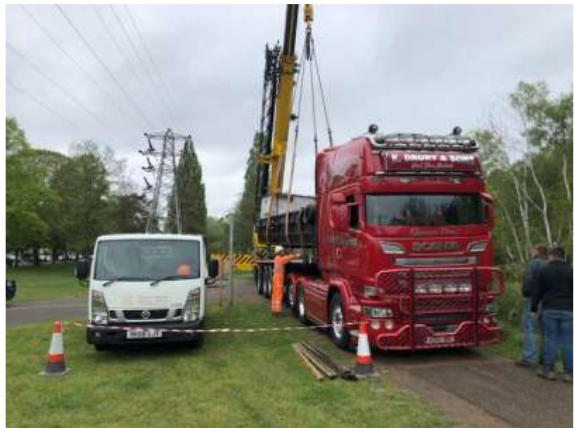
Boat almost in place, by River & Canal Services truck.
