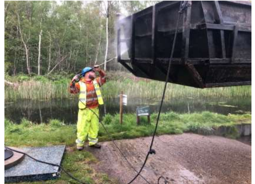
Aaron starts pressure-washing – a very wet job.
