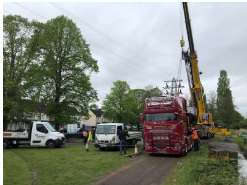
Loading complete at Woking. Note the electricity pylon.
