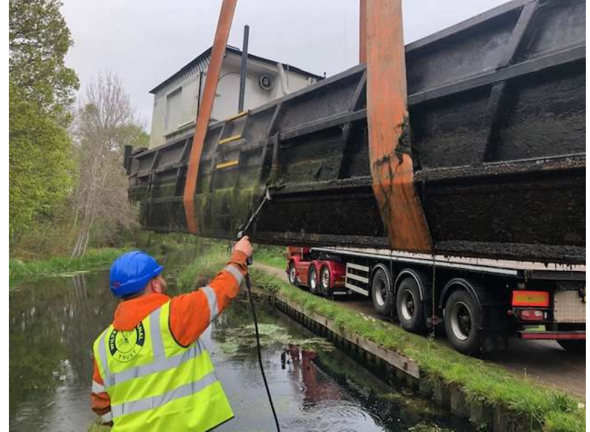
Starboard side half-complete.
